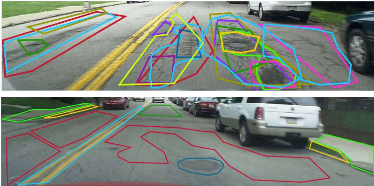
Figure 6 - Top: Positive labels (road cracks) as drawn by multiple annotators,
